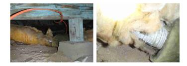
The ducts are a rigid metal type insulated with fiberglass. However, one of them is separated at near the middle of the home, and should be examined for evidence of rodent intrusion, and then reconnected and secured.
