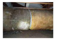
There is a PVC line connected to the main sewer line that could allow harmful gases into the interior circulating air. This is a health and safety hazard and should be removed.
