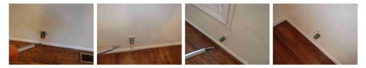
All most all of the outlets in the home are ungrounded and have three pronged outlets installed - Continued
