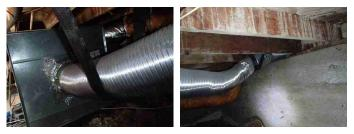
The return-air compartment needs to be sealed to prevent it from pulling crawlspace air and lowering the unit efficacy.
