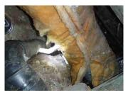
A terminated duct under the home is leaking air at the end of it and should be sealed correctly by a specialist.
