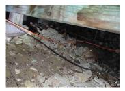
There is an electrical wire that is exposed that should terminate in an electrical junction box
