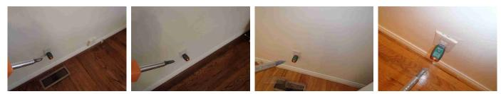
All most all of the outlets in the home are ungrounded and have three pronged outlets installed. This allows you to plug in electrical components that by today's regulations are required to have grounds. This condition should be evaluated and a ground fault circuit interrupter breaker should be installed on each circuit in the main electrical panel.
