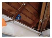
There are outlets hanging by the wires and exposed electrical wiring that should be addressed by an electrician for electrical safety reasons.
