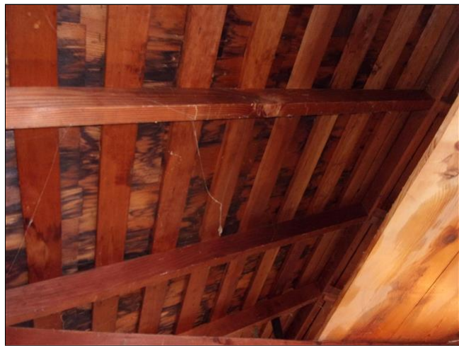
1.0 Item 2(Picture) asphalt shingles were installed over wood shake
