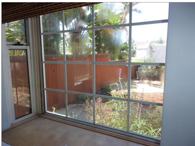
4.5 Item 1(Picture) possible evidence of dual pane seal defect observed
