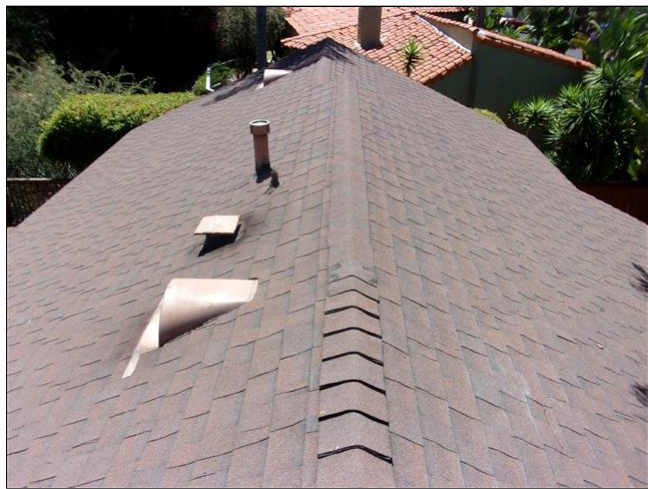
1.0 Item 1(Picture) recommend further evaluation of asphalt shingles over wood shake
