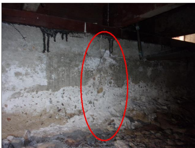
5.0 Item 7(Picture) cracks visible at the foundation stem wall / efflorescence observed
