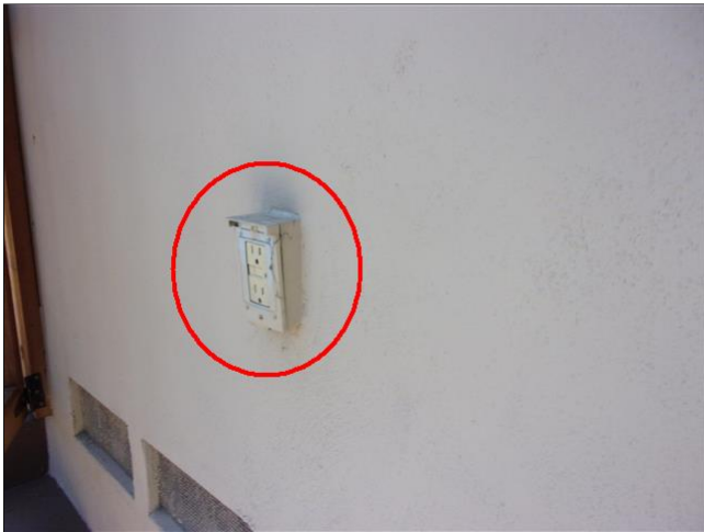
7.5 Item 7(Picture) missing outlet cover
