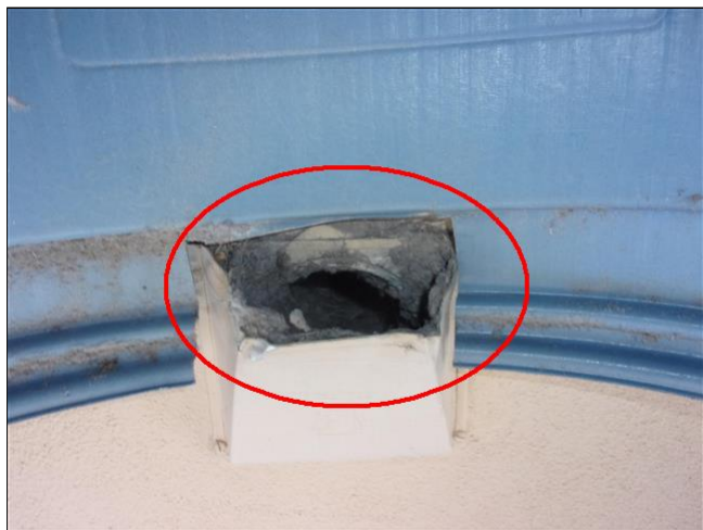
9.1 Item 1(Picture) dryer vent cleaning / maintenance/ repairs needed
