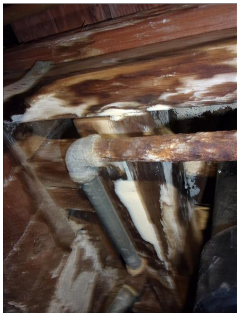
5.2 Item 1(Picture) below bathroom: moisture stains or damage visible
