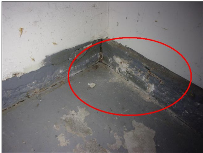
3.3 Item 1(Picture) efflorescence observed (drip irrigation observed at adjacent side of garage wall)
