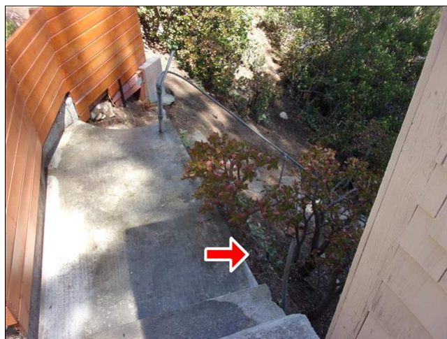
2.3 Item 2(Picture) fall hazard / railing safety upgrades recommended
