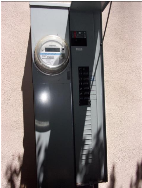
7.2 Item 1(Picture) electric meter and main panel
