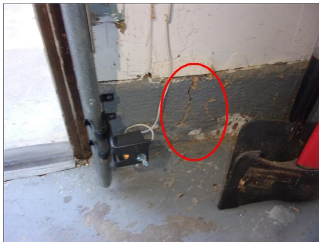
5.0 Item 2(Picture) cracks observed at garage foundation stem wall
