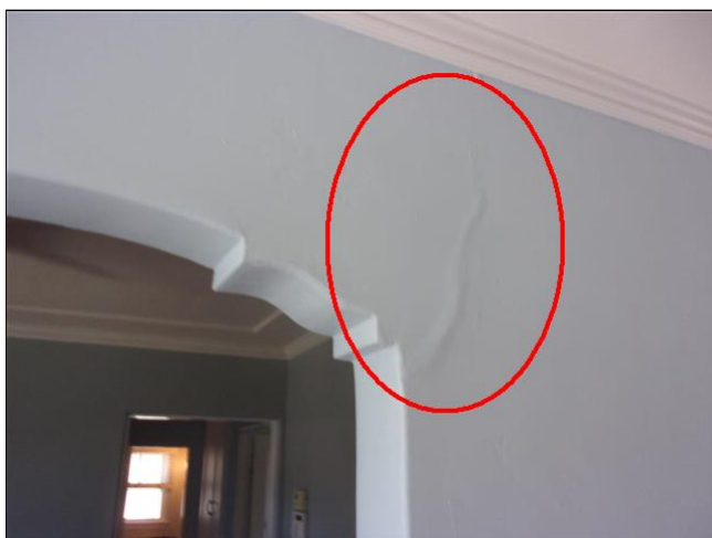
4.0 Item 1(Picture) cracks visible at interior wall
