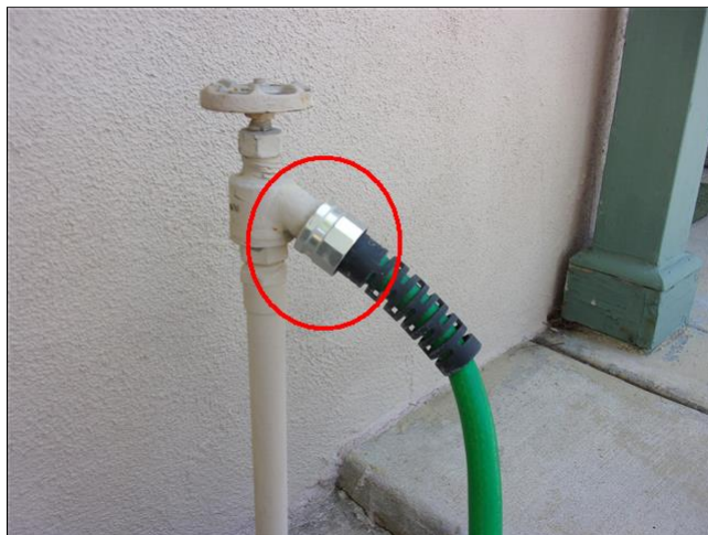
6.4 Item 2(Picture) aged water supply valves/hoses observed
