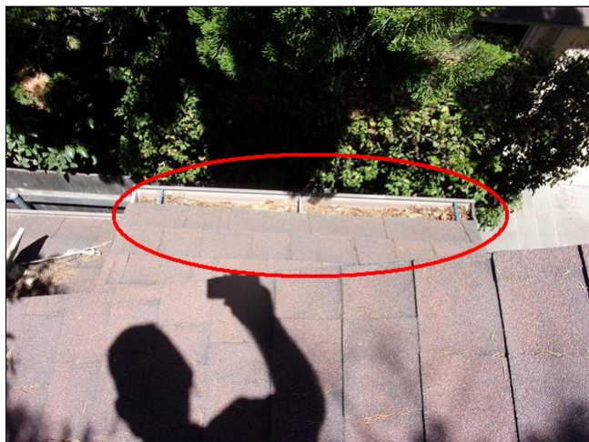
1.1 Item 3(Picture) rain gutter cleaning needed
