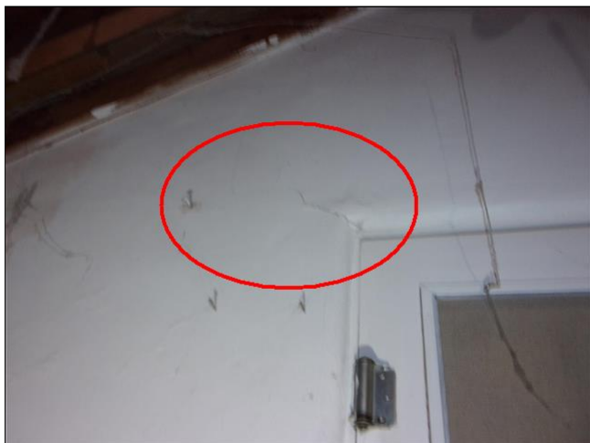
3.2 Item 1(Picture) cracks in garage wall observed
