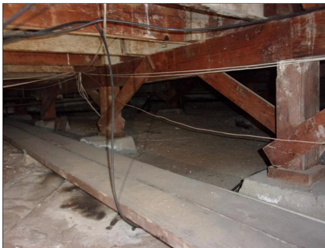
5.1 Item 2(Picture) post and pier seismic strapping/ anchoring upgrades recommended
