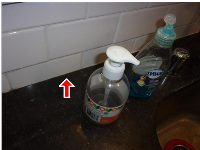
4.4 Item 1(Picture) kitchen: caulking or appropriate sealant maintenance/repairs needed
