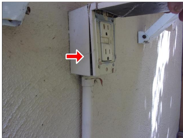
7.5 Item 2(Picture) exterior: loose outlet
