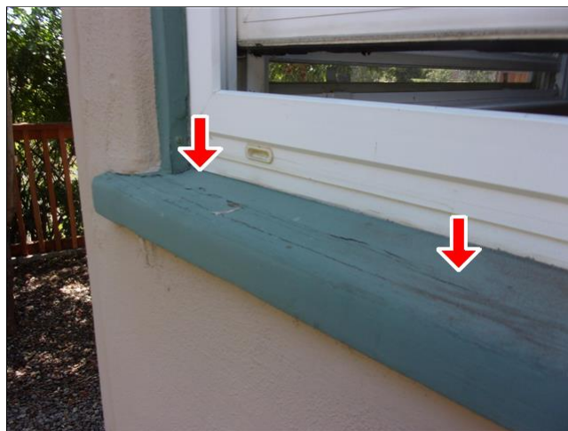
2.2 Item 3(Picture) window sill/trim: paint maintenance/repairs needed
