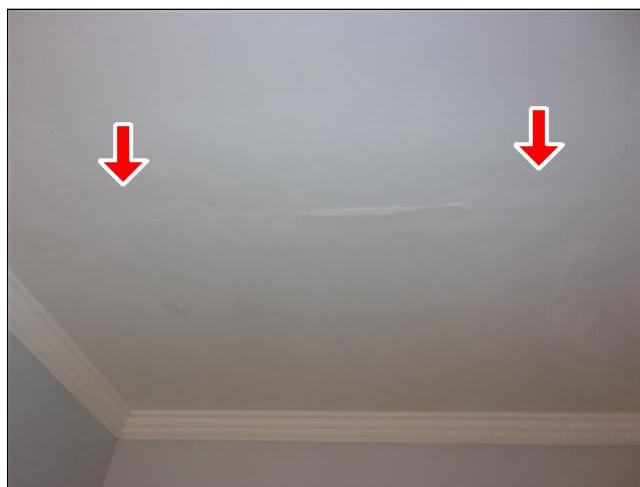
4.0 Item 2(Picture) cracks visible at bathroom ceiling
