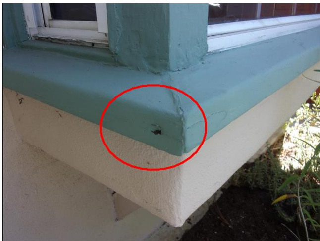
2.2 Item 1(Picture) near entry: possible WDO evidence or damage observed
