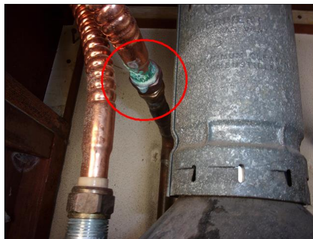
6.4 Item 4(Picture) near water heater: leaking observed at water supply
