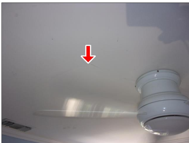
4.0 Item 3(Picture) cracks visible at bedroom ceiling
