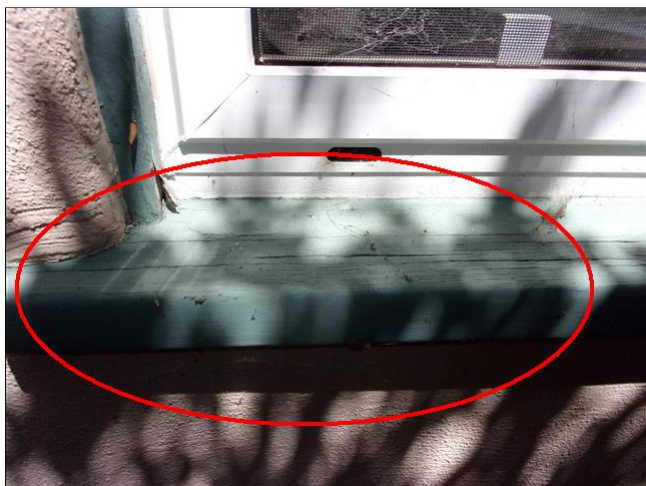
2.2 Item 2(Picture) window sill/trim: paint maintenance/repairs needed
