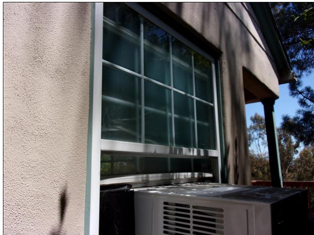
2.2 Item 4(Picture) possible evidence of dual pane seal defect observed
