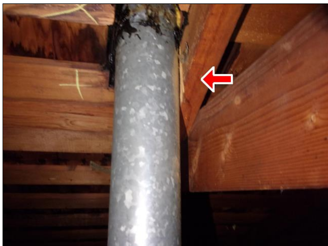
8.2 Item 2(Picture) FAU gas vent is in contact with combustible wood (2" minimum separation needed)
