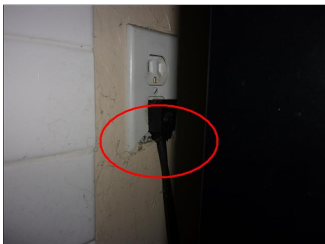
7.5 Item 3(Picture) kitchen: outlet cover maintenance/ repairs needed
