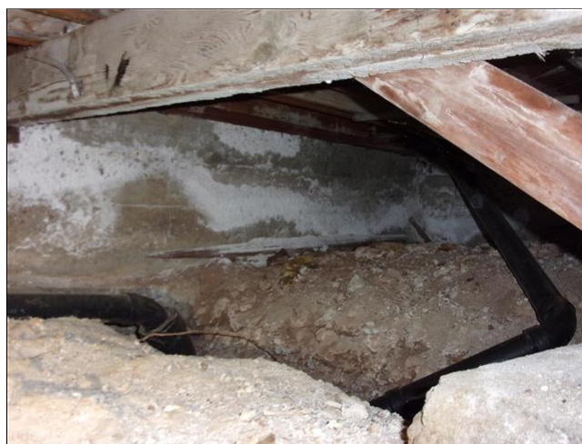
5.0 Item 4(Picture) efflorescence observed at the foundation stem wall
