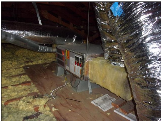
8.2 Item 1(Picture) attic FAU: no visible maintenance record observed
