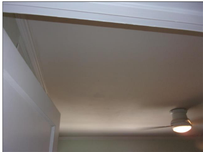
7.7 Item 3(Picture) missing bedroom smoke detector
