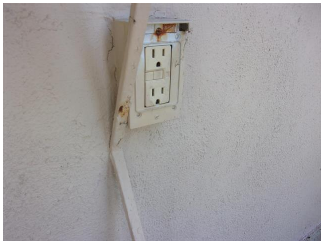
7.5 Item 1(Picture) missing exterior outlet cover
