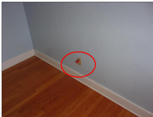
7.6 Item 3(Picture) reversed polarity observed when outlet was tested
