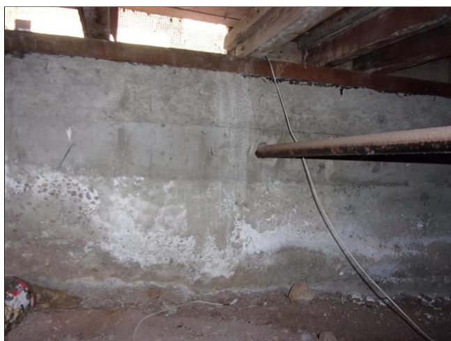
5.0 Item 3(Picture) efflorescence observed at the foundation stem wall
