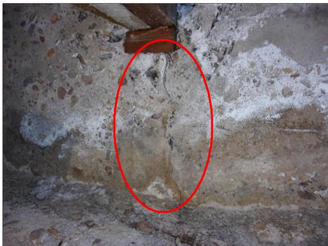
5.0 Item 5(Picture) cracks visible at the foundation stem wall
