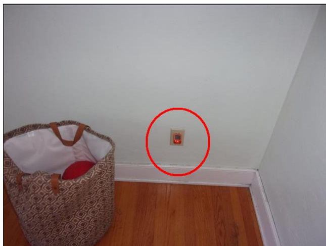
7.6 Item 2(Picture) reversed polarity observed when outlet was tested
