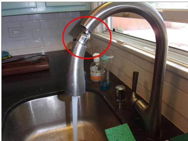
6.5 Item 1(Picture) kitchen: faucet leaked during testing
