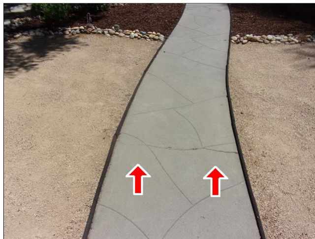
2.4 Item 2(Picture) crack in walkway
