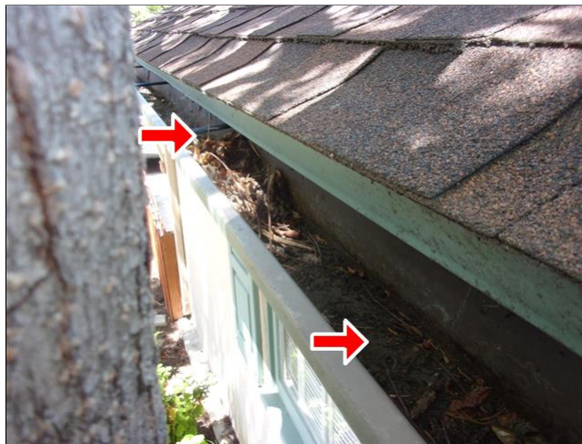
1.1 Item 2(Picture) rain gutter cleaning needed
