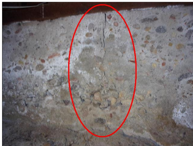
5.0 Item 6(Picture) cracks visible at the foundation stem wall
