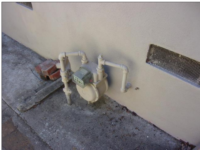
6.2 Item 1(Picture) gas meter and shut-off valve
