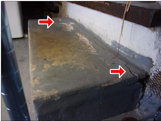
3.3 Item 3(Picture) cracks visible at garage step
