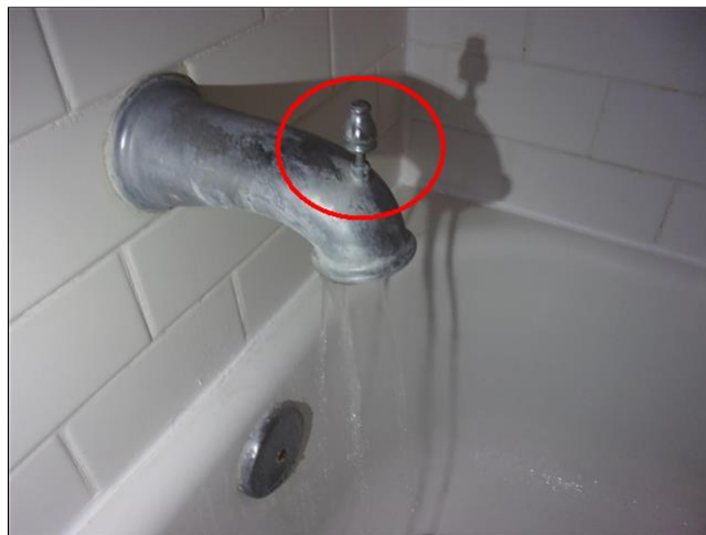
6.5 Item 2(Picture) tub spout diverter did not operate properly when tested
