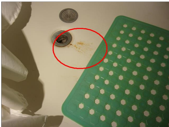
4.6 Item 1(Picture) oxidation visible at tub surface
