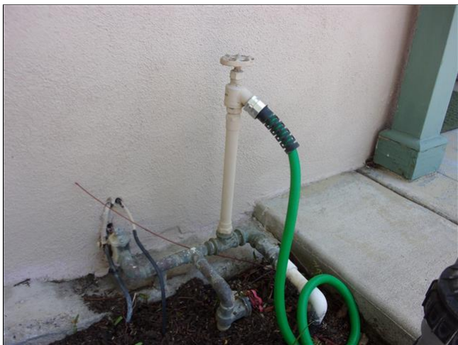
6.1 Item 2(Picture) house water shut off valve
