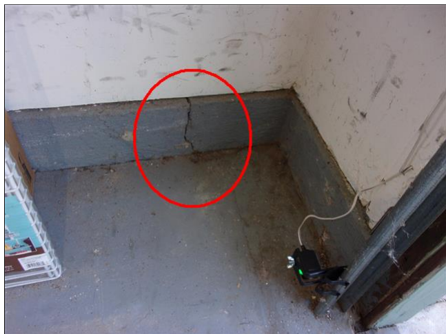
5.0 Item 1(Picture) cracks observed at garage foundation stem wall
