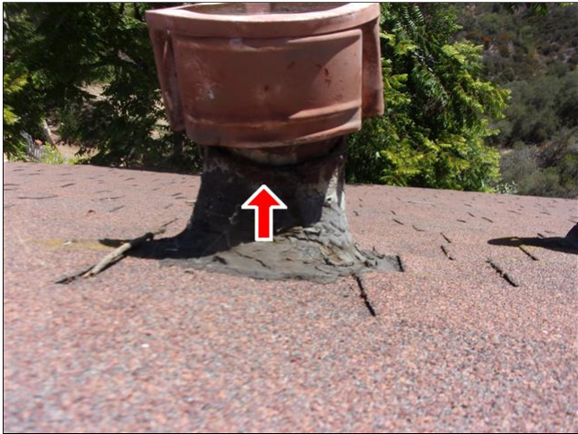
1.2 Item 1(Picture) boot flashing sealant separation visible
