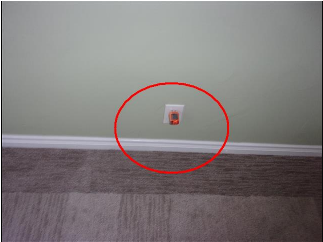
2.8 Item 6(Picture) non-grounded three-pronged outlets observed
