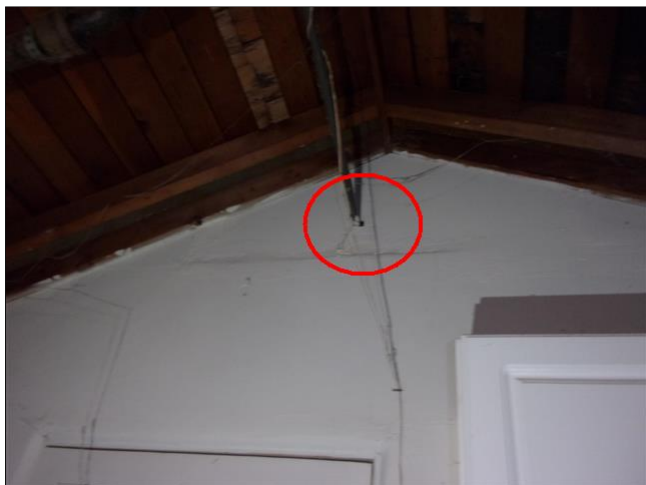
3.1 Item 1(Picture) penetrations observed in garage firewalls
